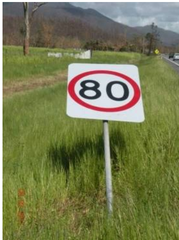
A failed road sign used to establish a lower limit of gust wind speeds in Cyclone 'Yasi'
