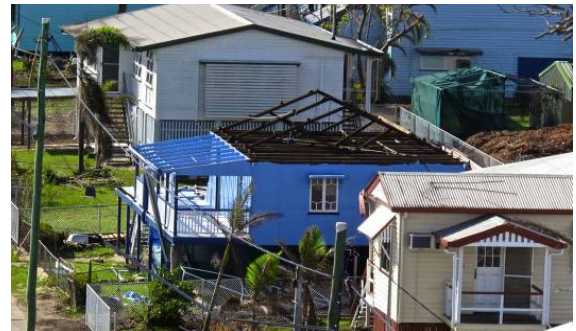
Damage suffered by pre-1980s houses during Cyclone 'Yasi'
