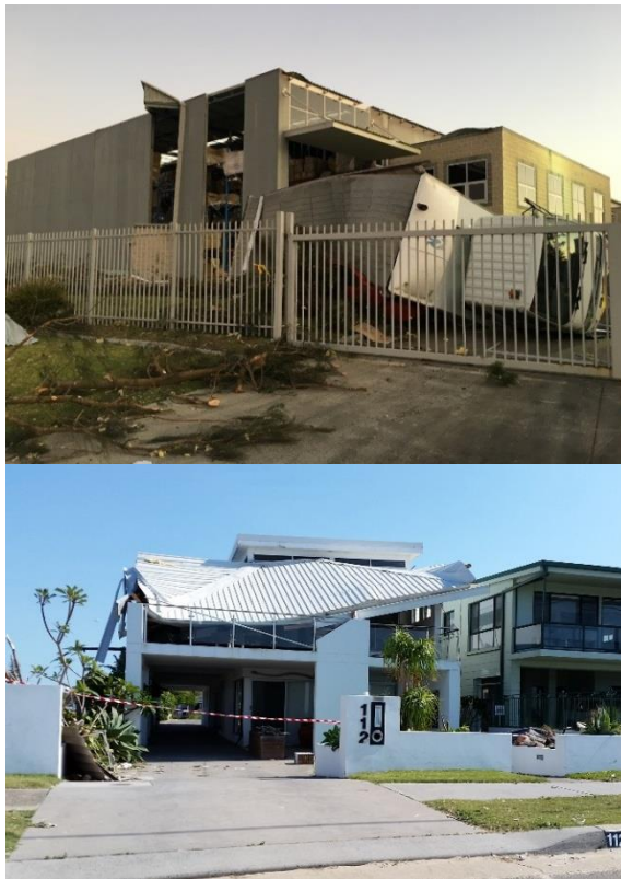
Figure 5. Examples of damage to industrial buildings (upper two) and residential buildings (lower two).
