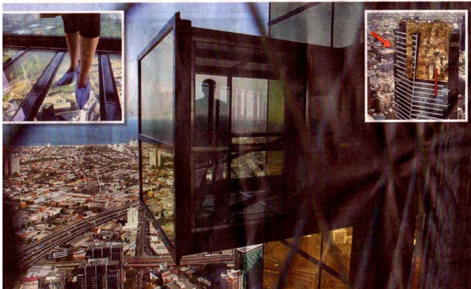
“The Edge”, a six tonne glass cube that juts out from the 88 th storey of the 92-storey Eureka Tower, 285m. Patrons can view the Melbourne skyline all year round, except when winds exceed 70km/hr.
