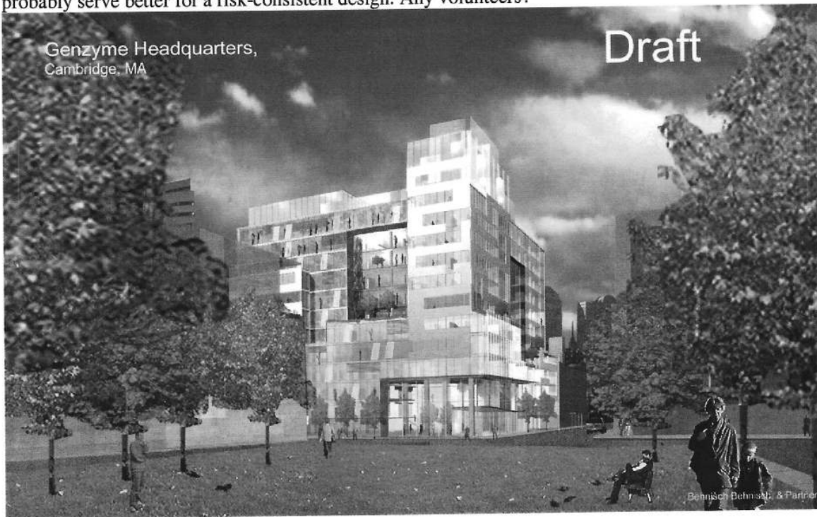
Figure 13: The Genzyme Headquarters in Boston, Massachusetts, was analyzed for cladding pressures when selected critical windows were assumed open during a design storm.
