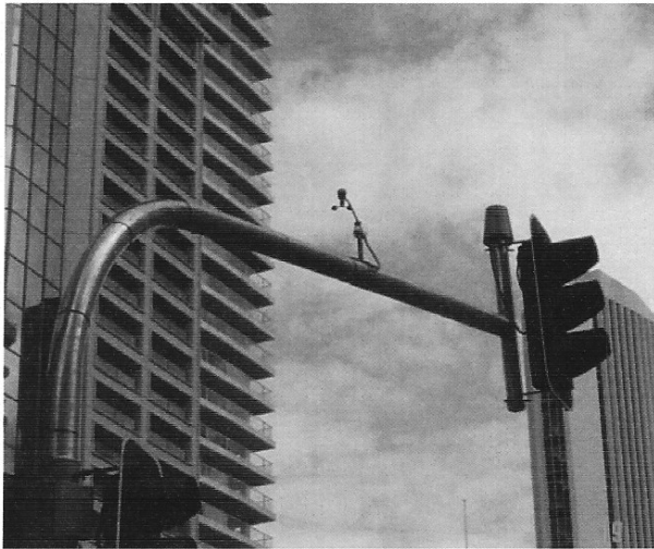
Fig. 2 Anemometer mounted on traffic light arm
