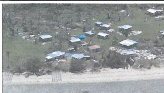
Figure 3: Damage caused by category 3 tropical cyclone Ami in Fiji, in 2003.
