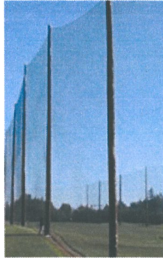
Figure 1: Very porous barrier netting is used around many sports facilities, such a golf course near a busy road (shown) or even on the roofs of tall buildings.
