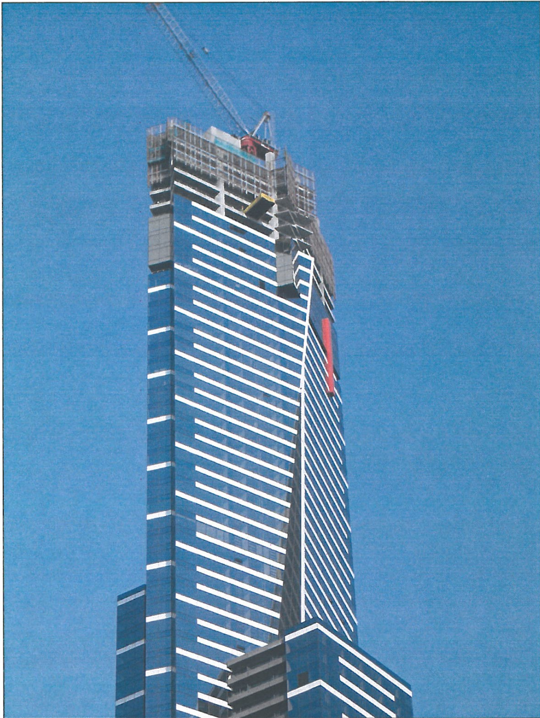
Figure 1D – Photo of approximate completion stage as at 30 th January 2006
