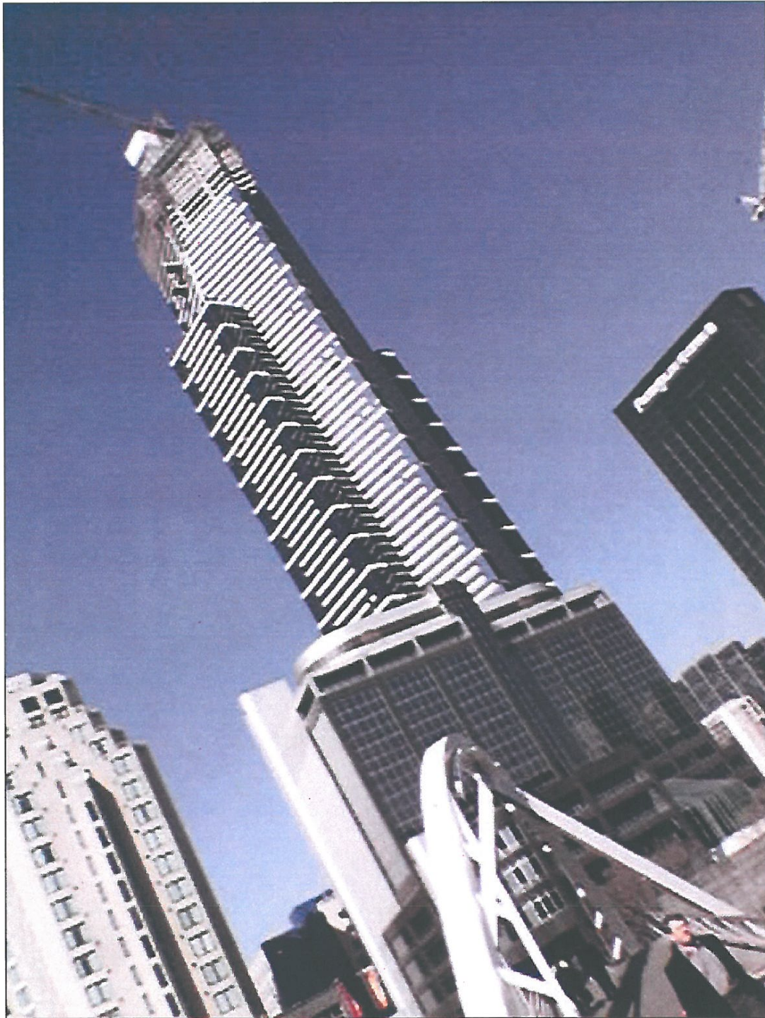
Figure 1B – Photo of approximate completion stage as at 25 th August 2005
