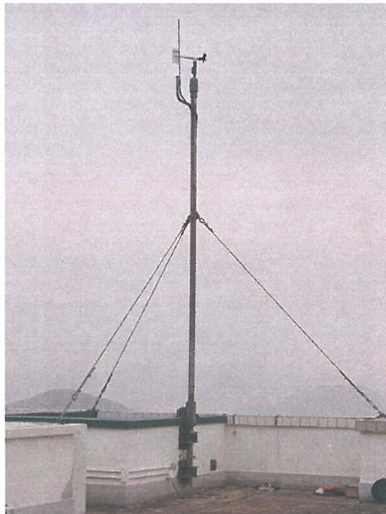
Figure 1 - The Mast on the Roof of Tower C, HKUST
