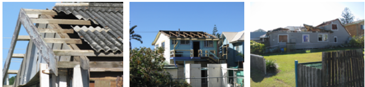
Enhanced Fujita scale EF0, 29-38 m/s Enhanced Fujita scale EF1, 39-49 m/s Enhanced Fujita scale EF2, 49-60 m/s
