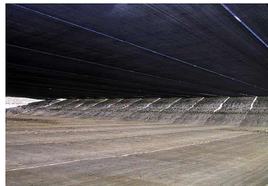
Figure 1b. Dam Cover Construction
