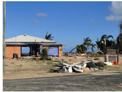
Figure 8. Single storey houses at Tully Heads - one washed away
