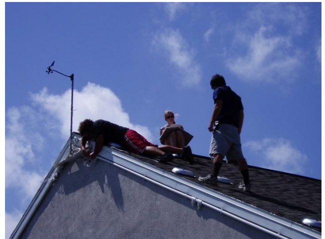
Figure 3. Installation of a FCMP house pressure measurement system
