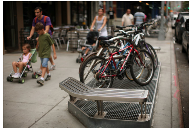
Figure 5. Giving the subway grates in New York City a bit more height will aid in the resilience against flooding from above (after Wilson, 2013).
