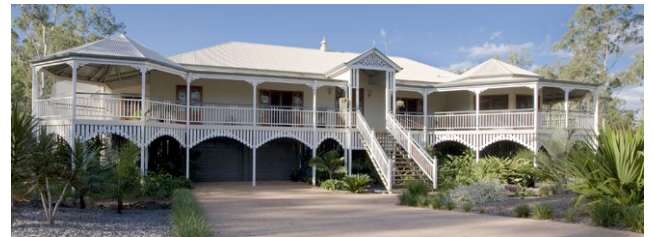
Figure 1. A typical elevated (to catch some breeze) home in Brisbane has a large wrap-around balcony (for shade). This architectural style is often generically referred to as a "Queenslander". This is potentially more resilient than the modern designs that rely on air-conditioning for comfort and livability.
