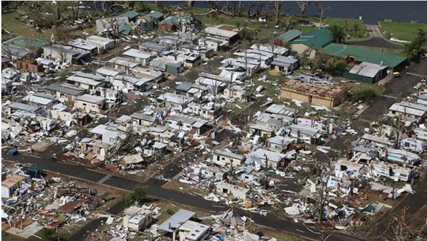
Figure 3. Aerial view of damage to the Denison County caravan park, Mulwala
