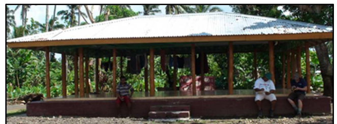
Figure 9. Typical Samoan Residential Fale, These buildings are a single storey open air with timber (or reinforced concrete) pylons connecting the roof structure with concrete slab or timber (piles) floor. Other typical features include a sheet metal or thatched roof.
