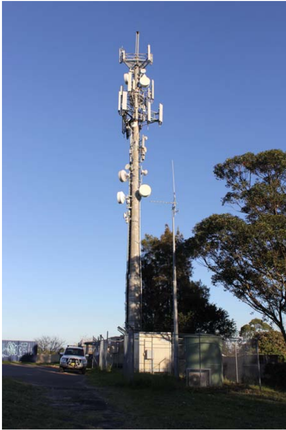
Figure 5. Monopole D prior to steel jacket installation (Test 1 Condition)
