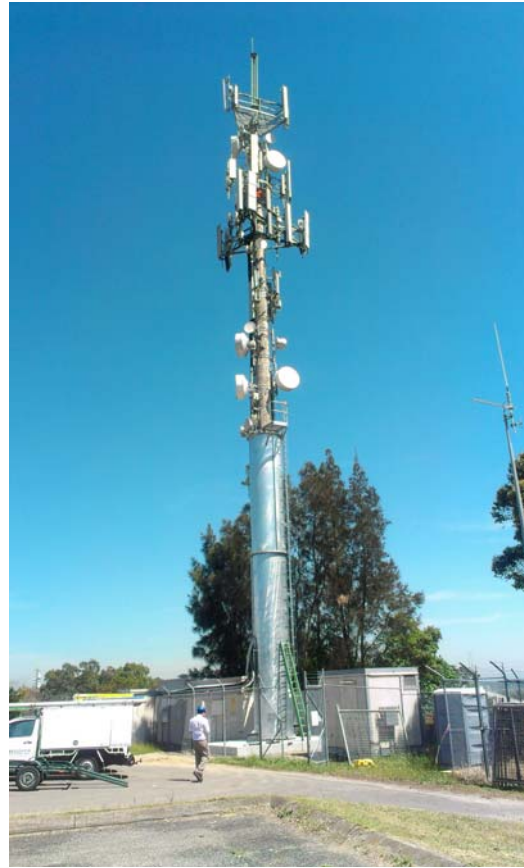
Figure 6. Monopole D after steel jacket installation (Test 3 Condition)
