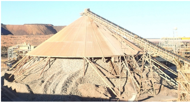
Figure 1. Example Ore Stockpile Cover.
