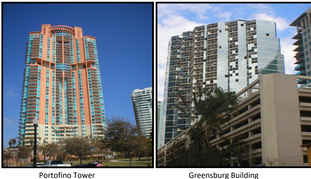
Figure 5: Portofino Tower vs Greenburg Building (Code vs no Code)
