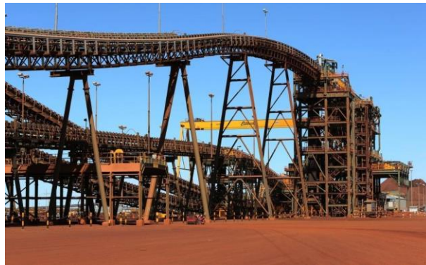
Figure 1. Typical iron ore handling plant showing conveyor and transfer tower
