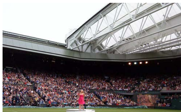
Fig 8 Wimbledon Centre Court Closing roof, first use.
