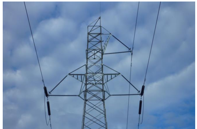
Figure 3: Towers with pivoting cross arms (modified)
