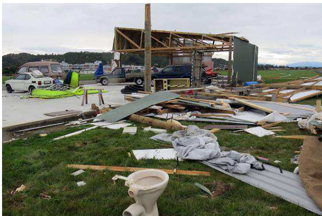
Figure 6. Aircraft hangar at Greymouth Airport destroyed.
