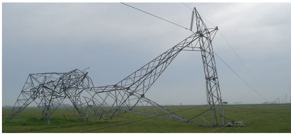
Figure 2: Failed tower on the investigated line following a downburst event in 2006.
