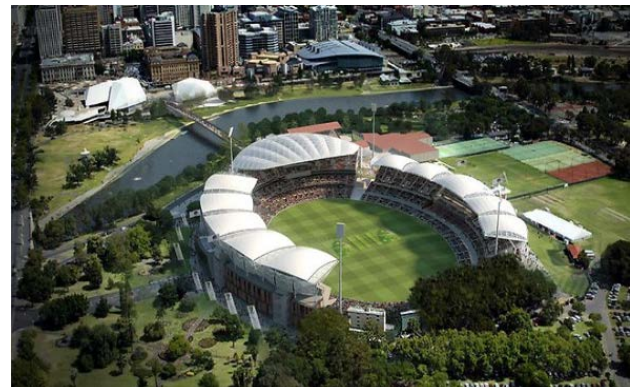
Figure 2 3D image of the completed Adelaide Oval Redevelopment
