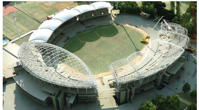
Figure 8 Diagrid roof structure
