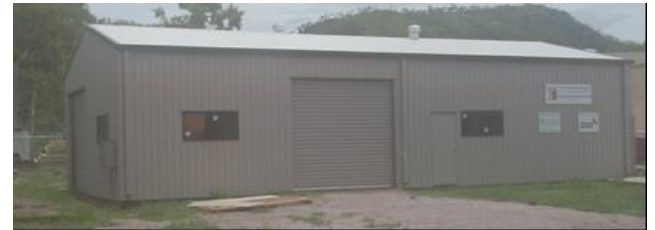
Figure 1. Full-scale Cyclone Testing Station test building
