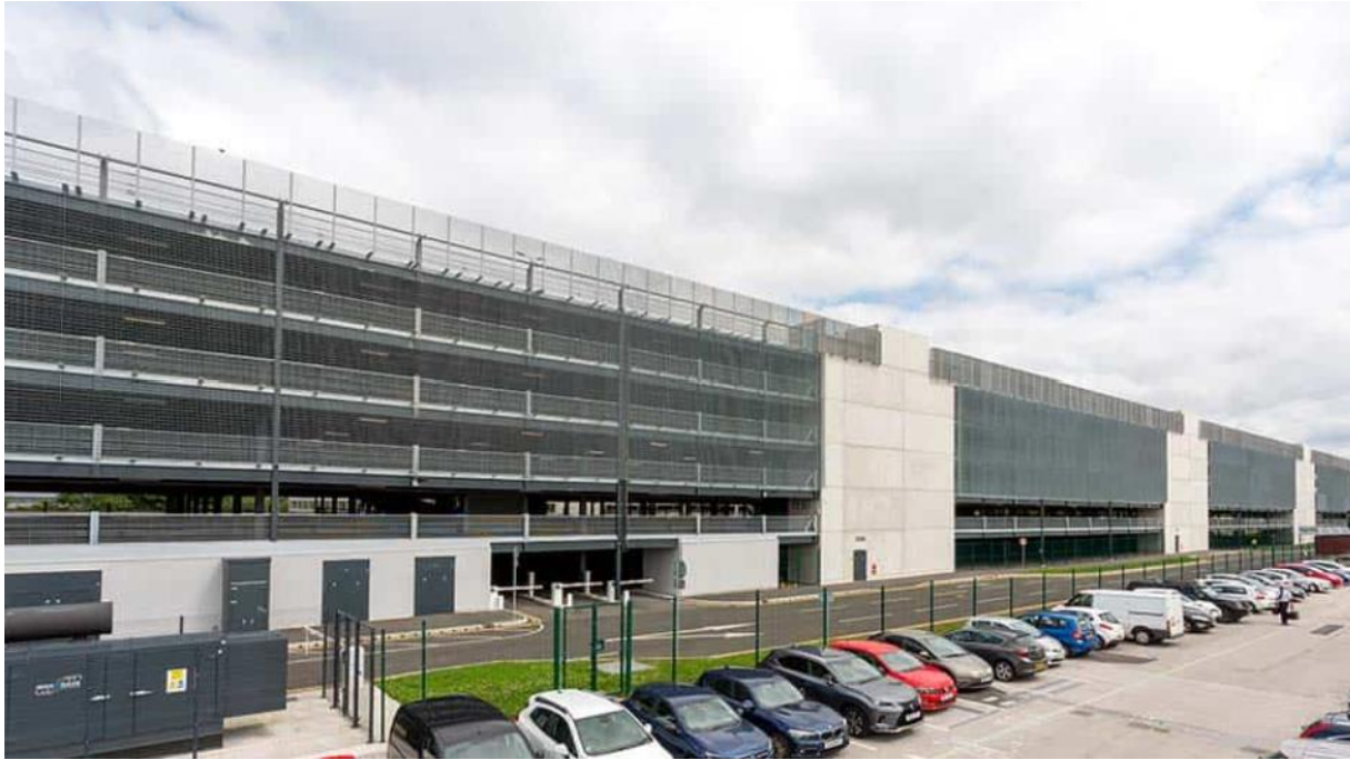
Figure 4. The second largest MSCP in Europe at Manchester Airport
