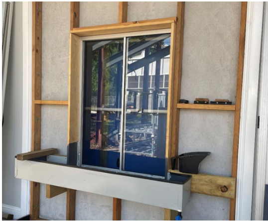
Figure 2 N3 Sliding window installed in the WDRI simulator.
