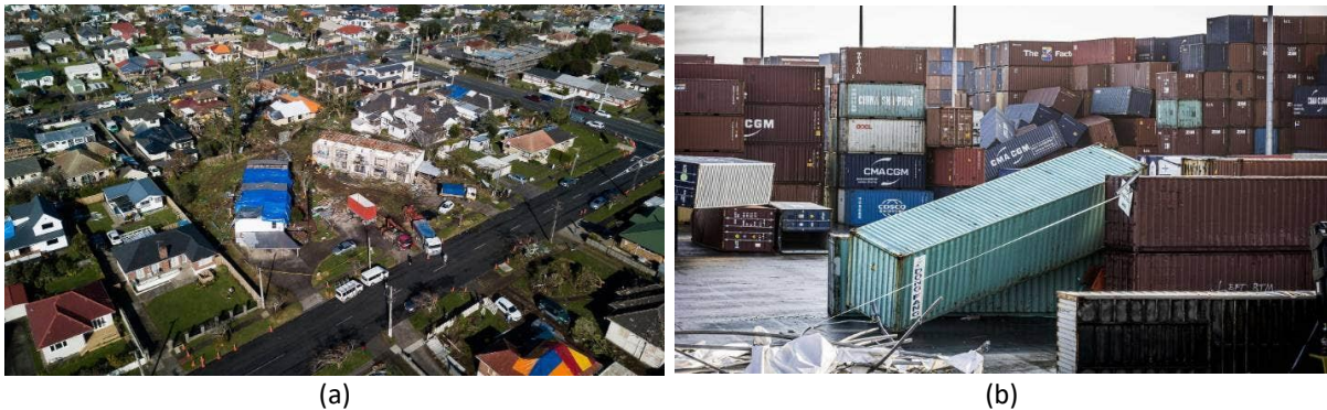
Figure 1. (a) Aerial image of the tornado damage in Papatoetoe, Auckland (Stuff, 2021). (b) Damaged shipping containers at the ports of Auckland, Wiri (Stuff, 2021).
