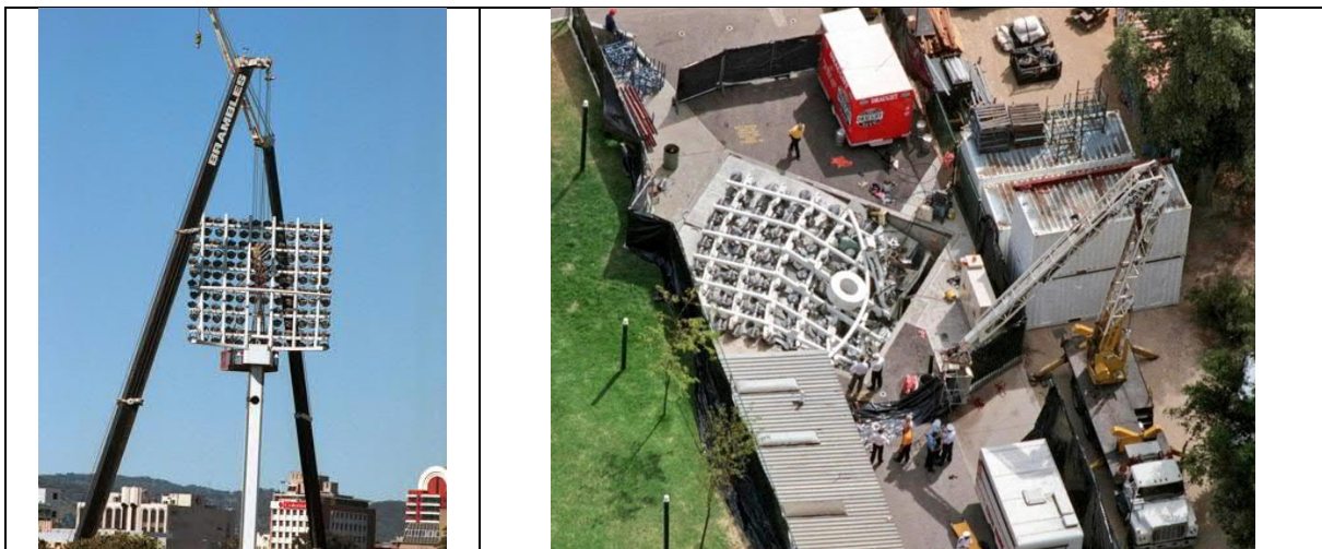
Figure 1 Original Adelaide Oval Light Towers
