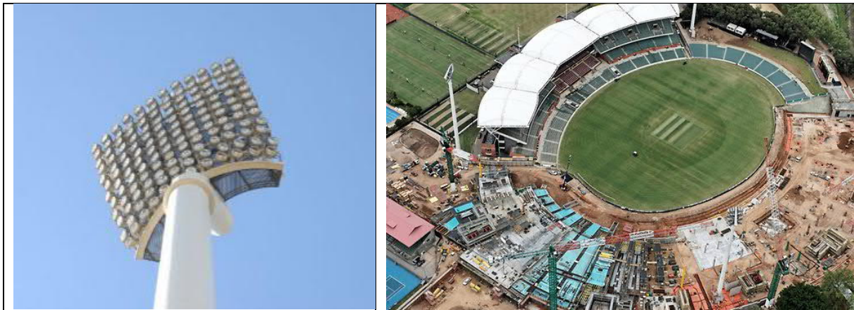
Figure 2 New light towers at Adelaide Oval integrated into the redevelopment
