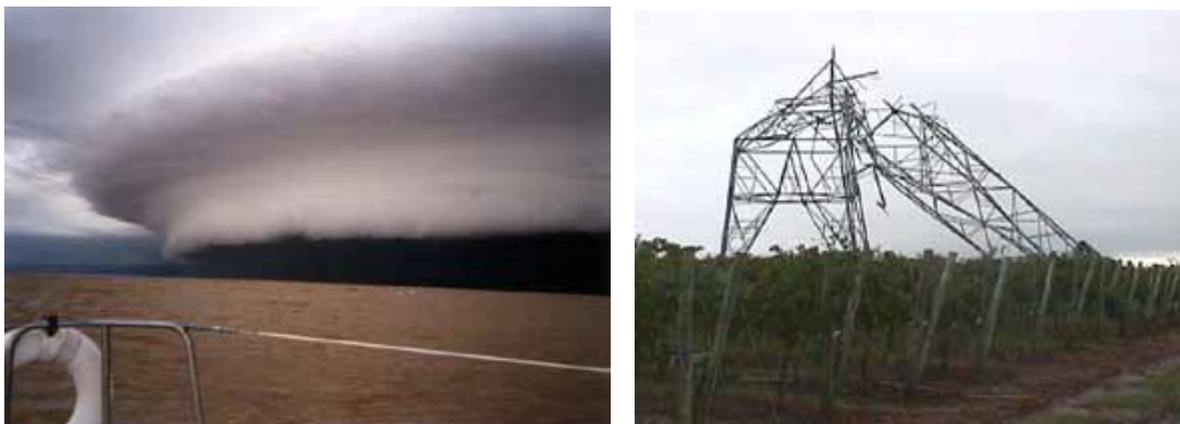
Fig. 3. Meso-cyclone in River Plate & damaged high transmission tower, March 10 th , 2002
